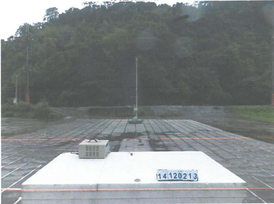
01 RE Front View
